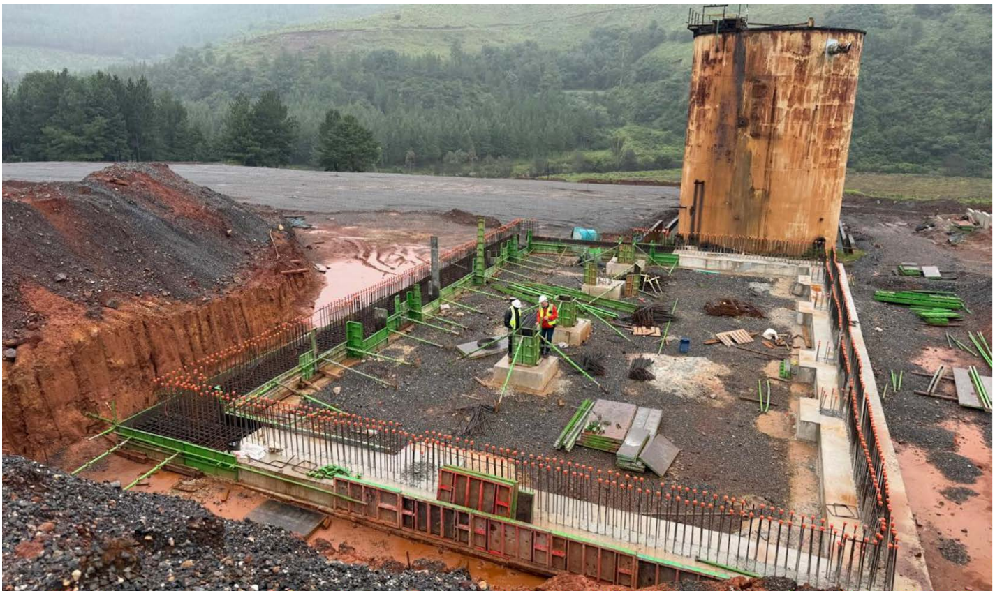
Figure 3: The Gold Room's Foundations
