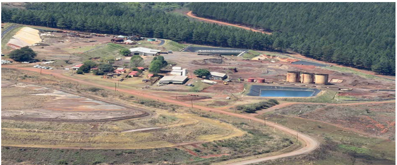
Figure 4: Aerial photo of the existing Plant post decommissioning of old facilities.
