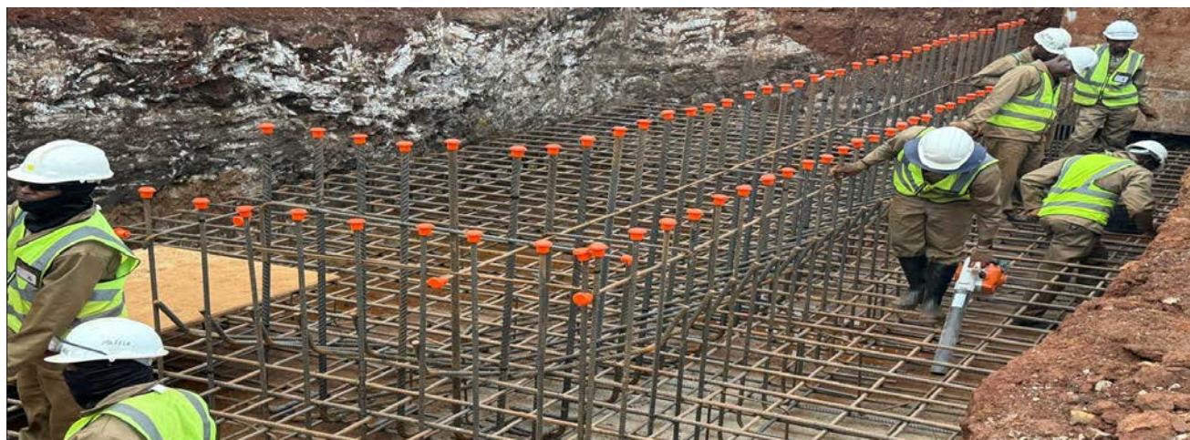
Figure 2: Steel reinforcing installation and preparation for concrete placement
